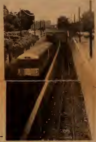
Rapid Transit commuter rails and Amtrak trains will run in a trench similar to this one north of Philadelphia, designed by F.R. Harris, Inc.
